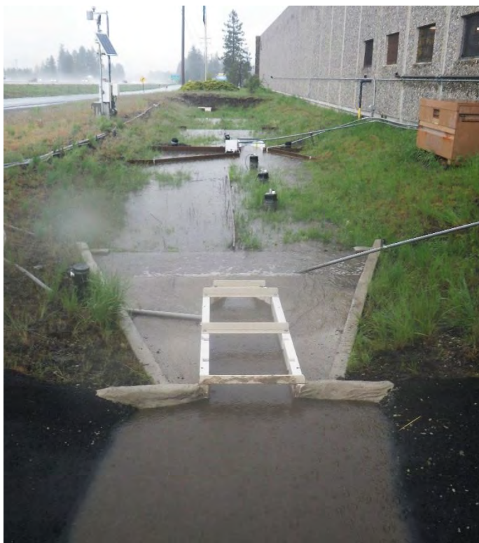
Figure 4. Example of a compost-amended biofiltration swale. Stormwater is filtered as it flows along the grass in the swale and infiltrates into the topsoil and compost. Photo: Washington State Department of Transportation.
